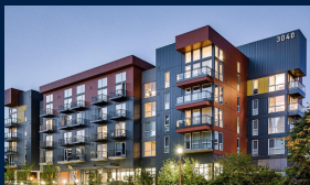
Multifamily | Redmond, WA $69 Million Senior
