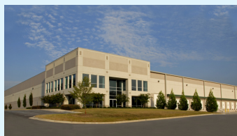
Industrial Portfolio | Nationwide $408 M Senior + Mezzanine
